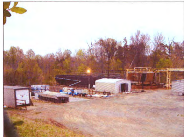
Northern area of the Custom Chemical facility
