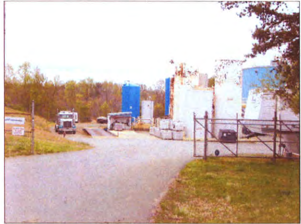
Main entrance into Custom Chemical – note the vertically positioned Aboveground Storage Tanks (ASTs) – view is to the east
