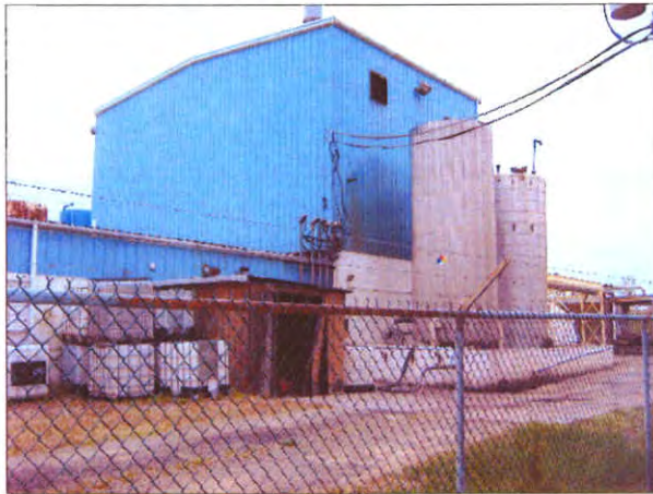
Eastern area of Custom Chemical facility – note the vertically positioned ASTs
