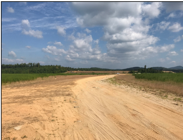
Northern view from the central area of the Site
