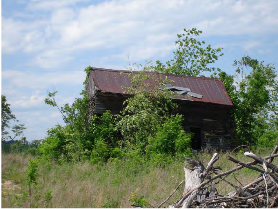
Plate 8. View of Structure #5, Barn, looking north.
