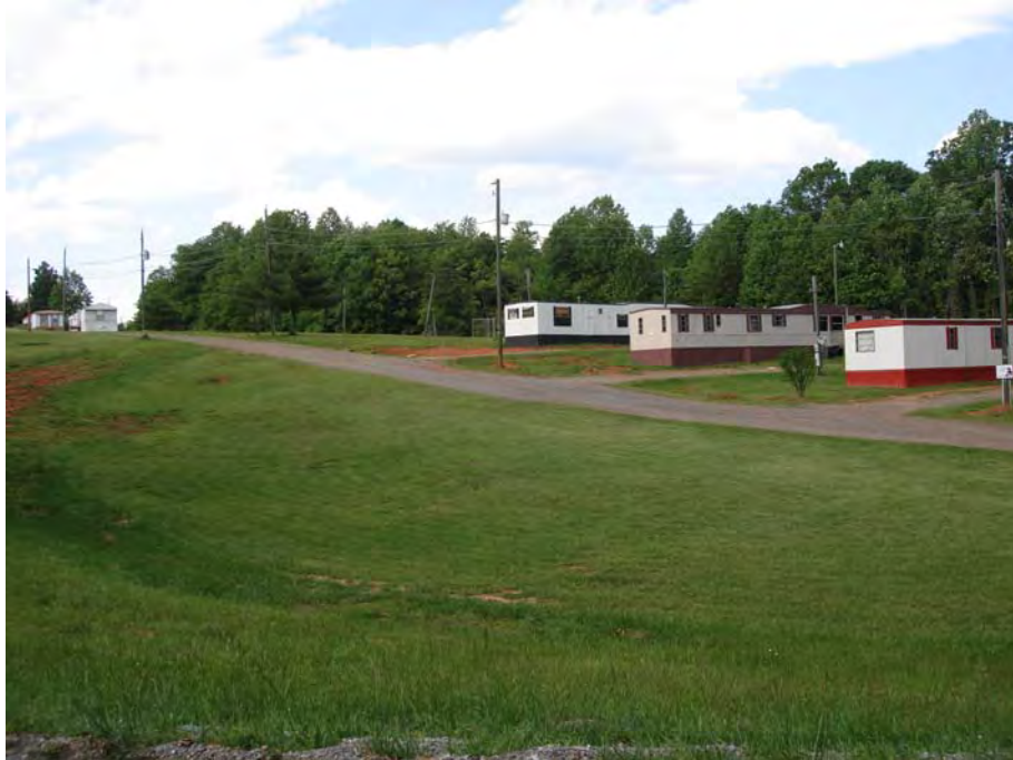
Plate 29. View of Adjacent Structure, Trailer Park looking southeast.
