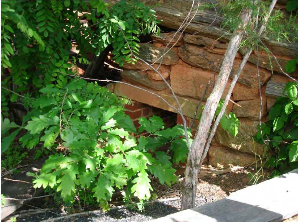
Plate 4. View of Structure #3, Barn, foundation detail.
