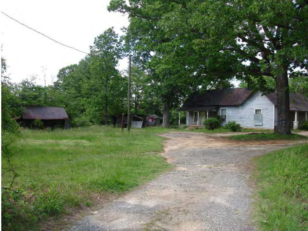
Plate 26. View of Structure #1, Single Dwelling and Barns, looking northeast.
