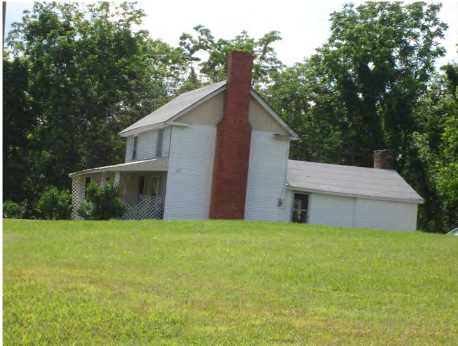
Plate 28. View of Adjacent Structure, Single Dwelling, looking north.
