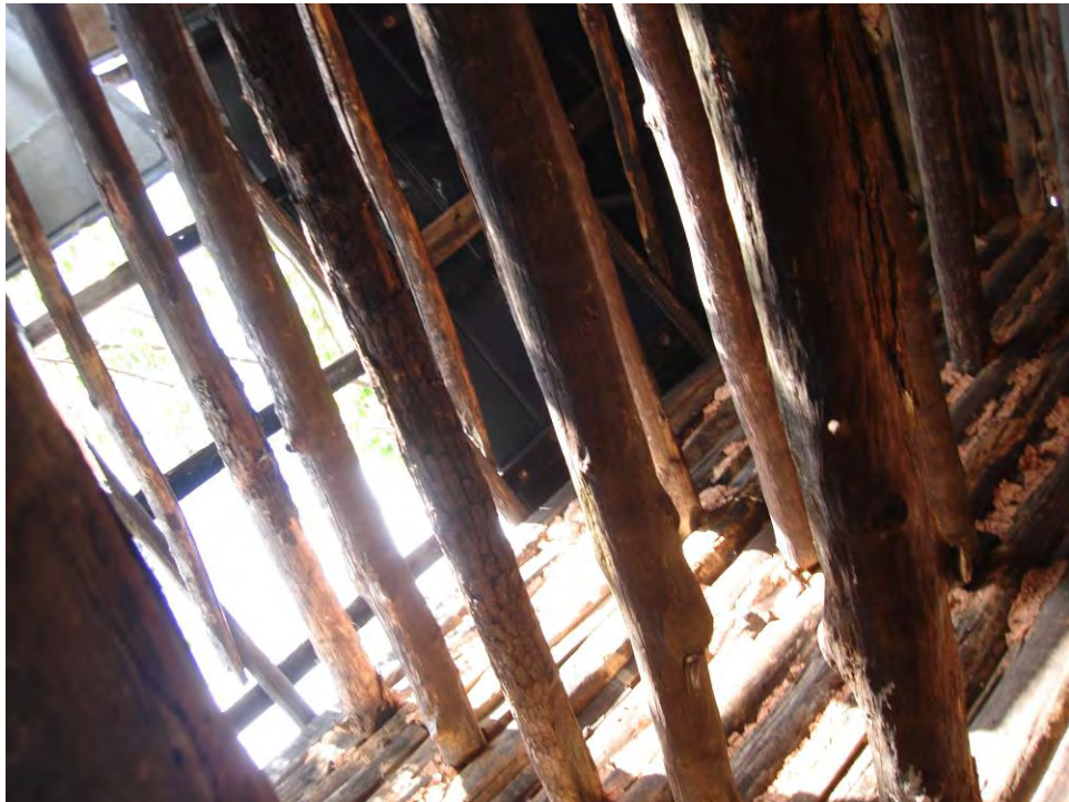
Plate 5. View of Structure #3, Barn, roof interior.
