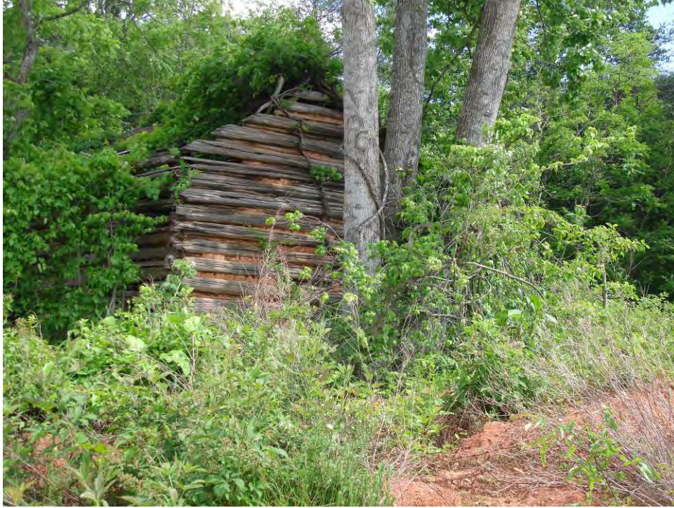
Plate 2. View of Structure #2, Barn, looking west.
