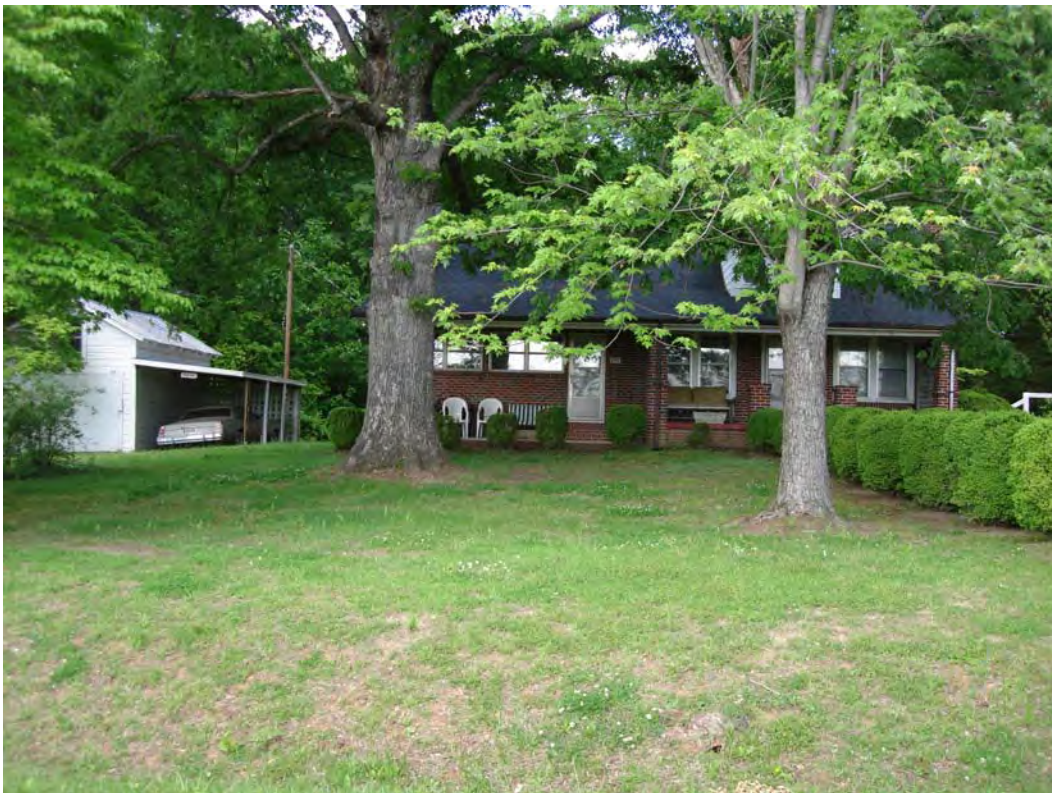
Plate 31. View of Adjacent Structure, Garage, looking east.
