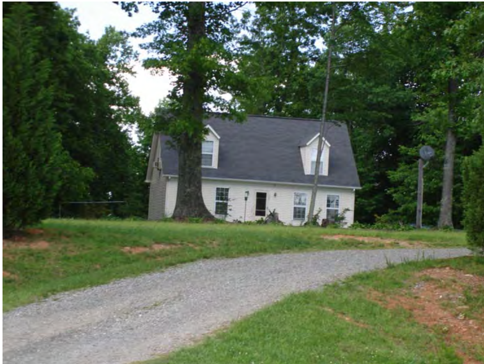
Plate 27. View of Adjacent Structure, Single Dwelling looking west.
