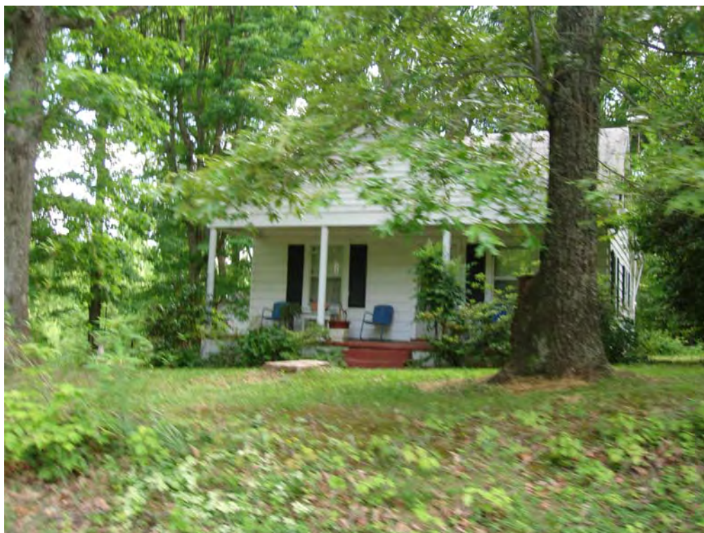
Plate 21. View of Adjacent Structure, Single Dwelling, looking west.
