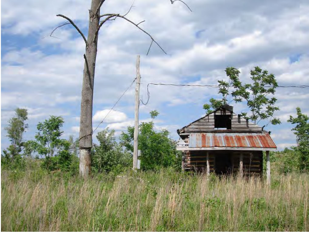
Plate 7. View of Structure #4, Single Dwelling, façade, looking east.
