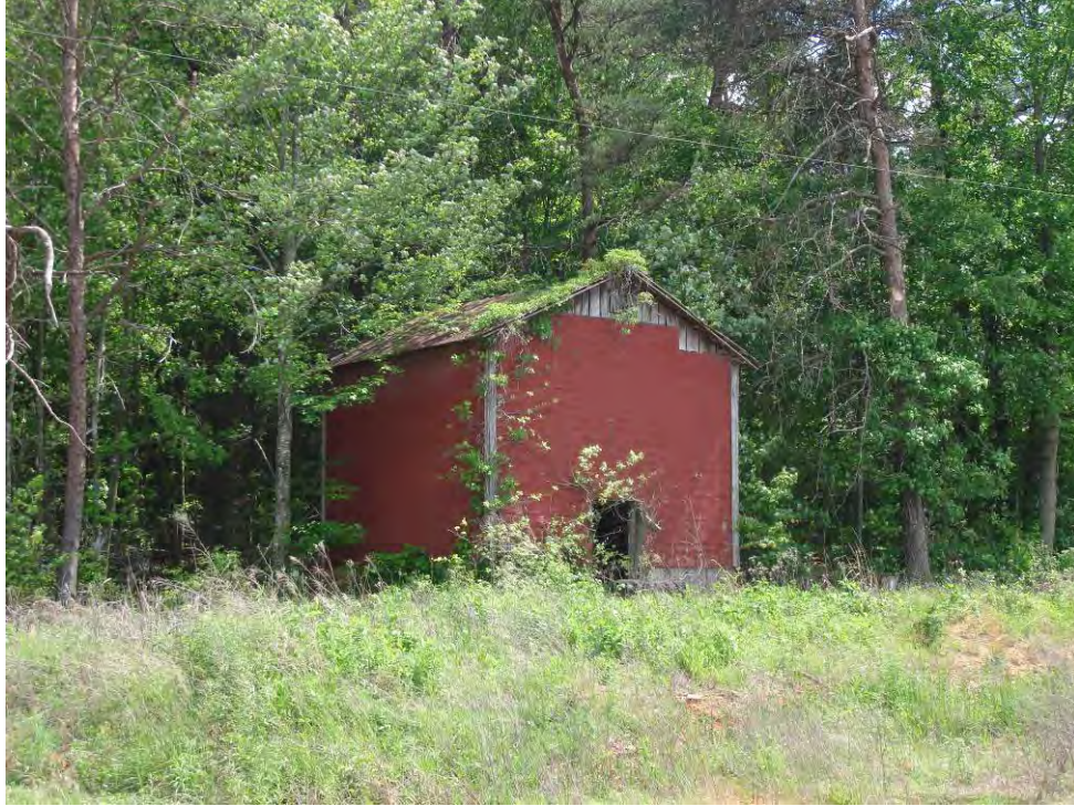
Plate 1. View of Structure #1, Barn, looking south.
