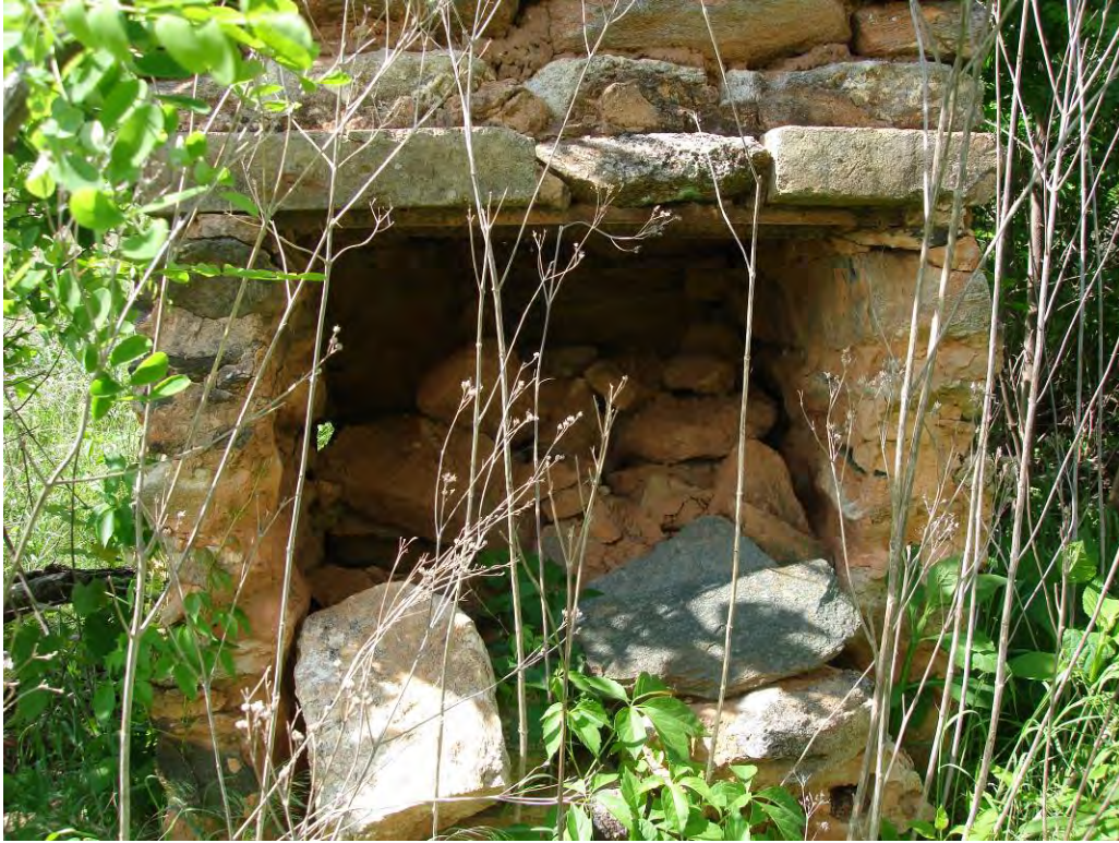
Plate 11. View of Chimney, base detail.
