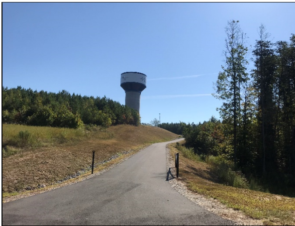
Water tower on the Site
