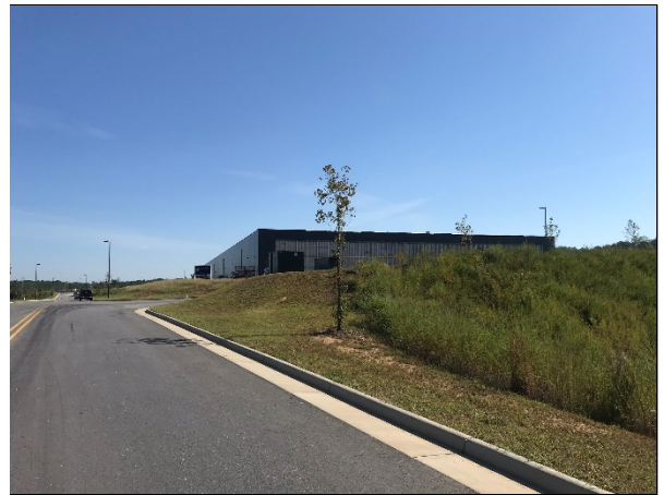
Under construction industrial facility on the Site
