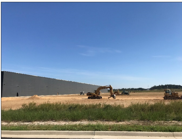
Under construction industrial facility on the Site
