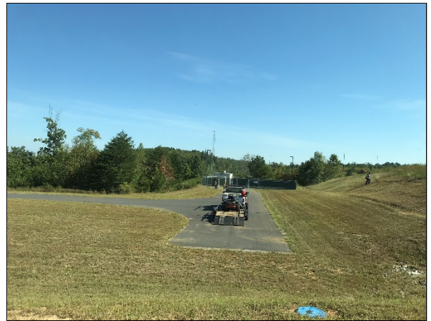
Pump station in the central area of the Site
